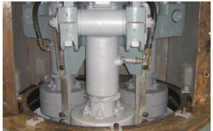
Mill with screens and covers removed.
