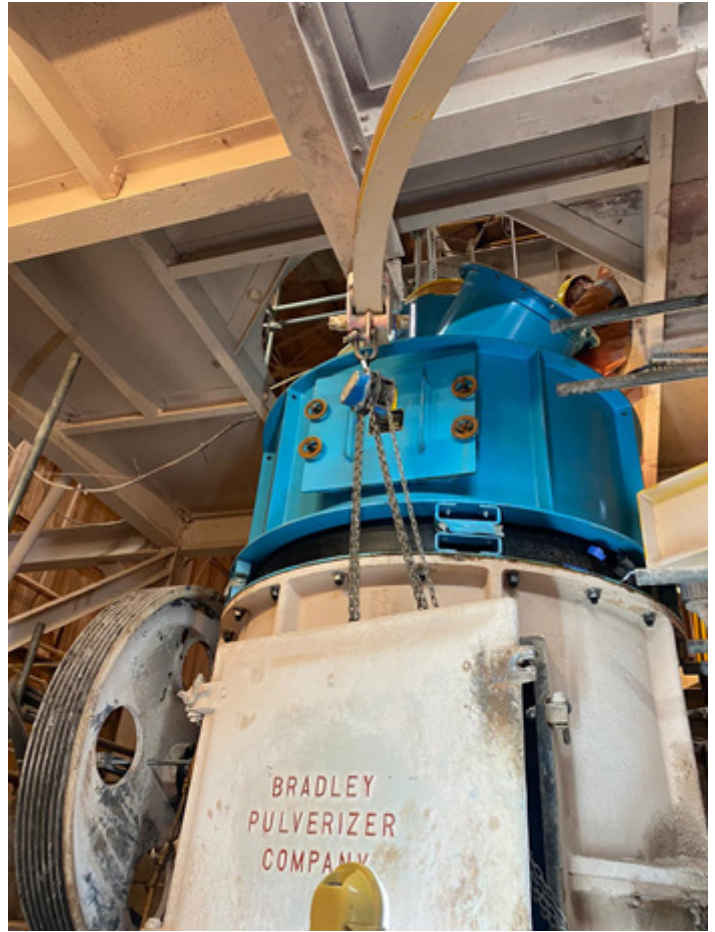
Figure 3: Completed mill overhaul with new VBC
