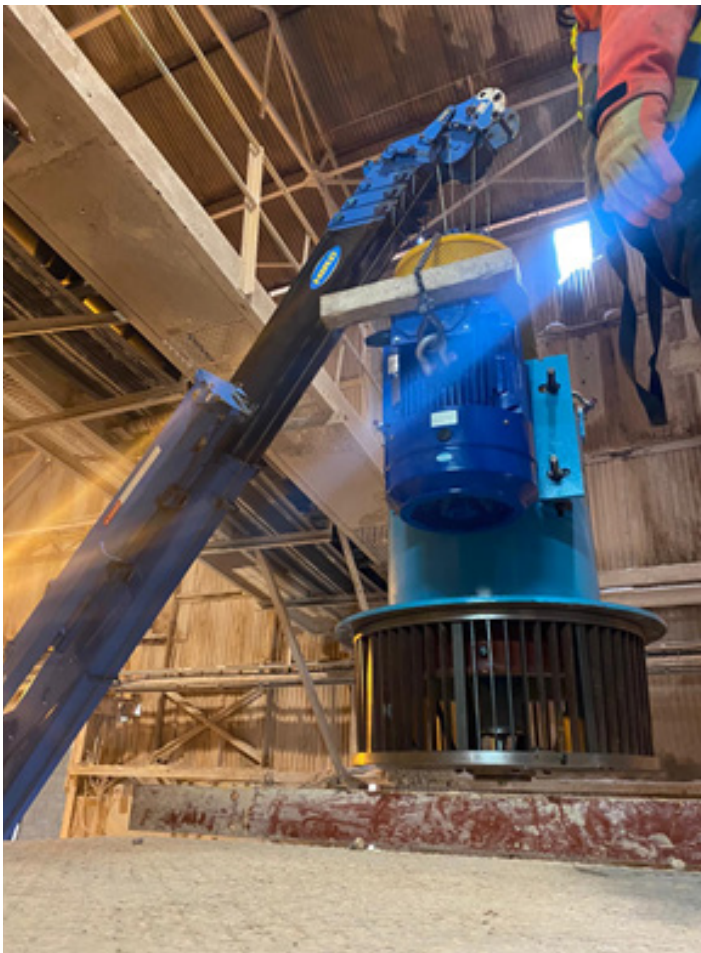
Figure 2: New VBC installation.
