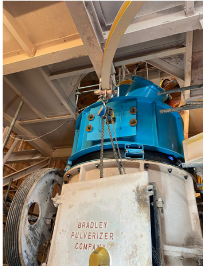
Figure 3: Completed mill overhaul with new VBC
